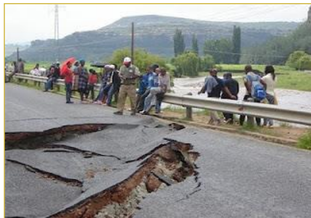
Collapsed infrastructure as a result of torrential rainfall in 2011
